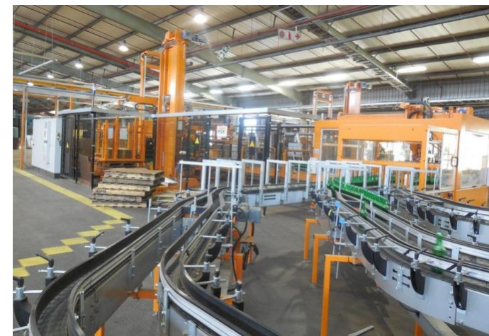
Furnace 3 cold end
